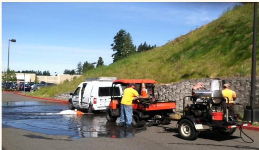
For the past few months, the Water Department staff has been flushing hydrants on the north end of the City. Fully operational fire hydrants are critical to municipal fire protection readiness. To ensure that hydrants will function correctly in response to fire emergencies, regular maintenance including flushing and inspection, cleaning, and painting must be performed.
