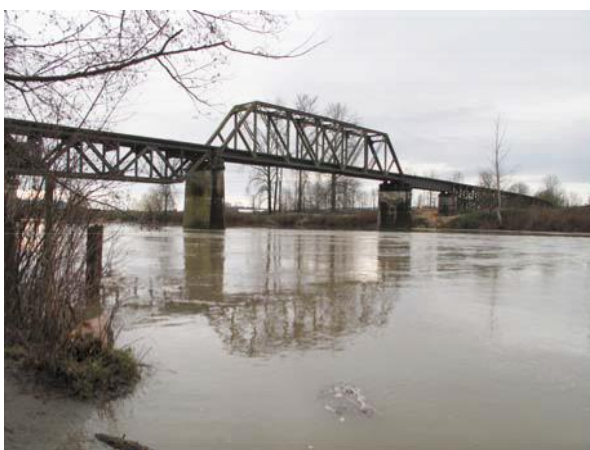
Railroad trestle bridge
