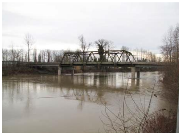
Avenue D bridge over Snohomish River
