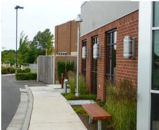
Parking lot lights, pedestrian scale lighting, and building lighting.
