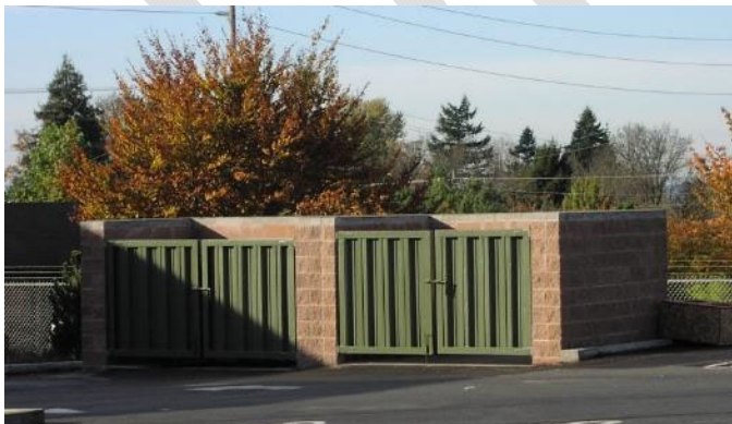
Masonry enclosure structure with metal gates.
